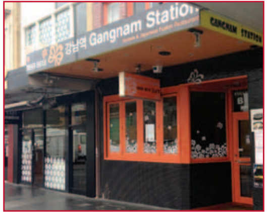
(After) Freshly painted window and door frames has brightened the shopfront against the contrast of the dark tiles. The new, consistently designed signs have dramatically improved the presentation of the shopfront.
