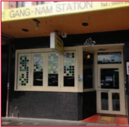
(Before) The shopfront was inconsistent in colour, signage and the window treatment was unprofessionally implemented. (Gangnam Station; Box Hill, VIC)
